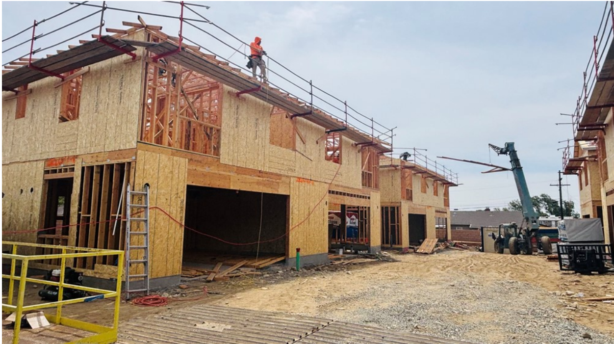
Washington Blvd Condominiums - 564-588 E. Washington Blvd (Under Construction) - August 2026
